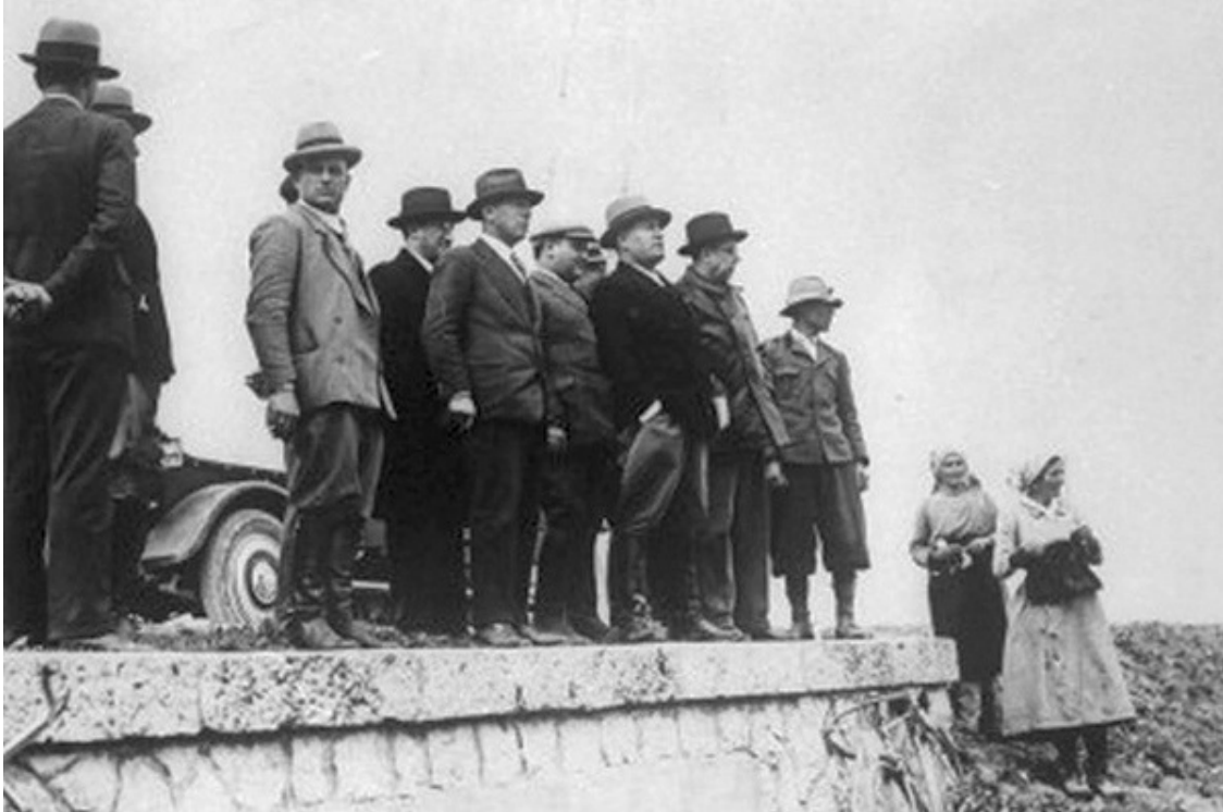
Mussolini inspects progress on the draining of the Pontine Marshes - one of his engineering triumphs which transformed this region into a thriving agricultural area.
